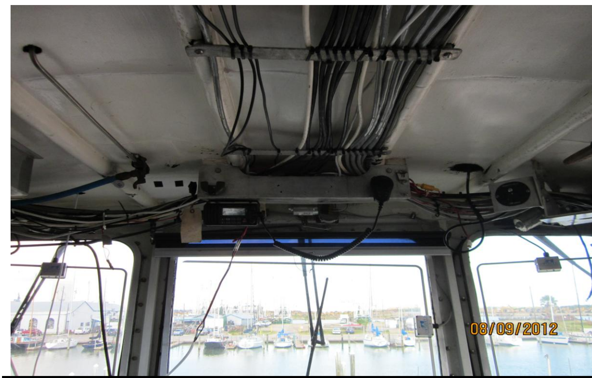
Photo 5, Panel for nav. Aids above pilot station.
